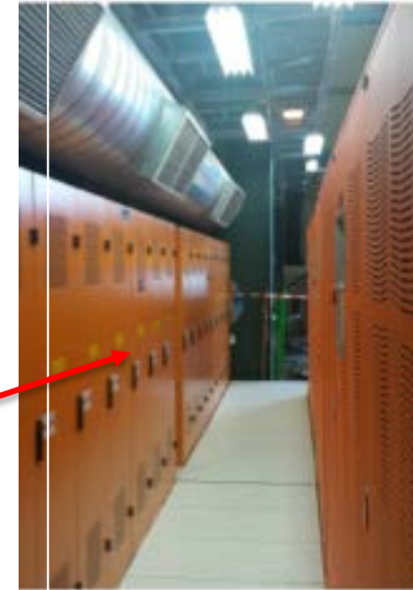
1MVA UPS in ATLAS SX1 surface building
