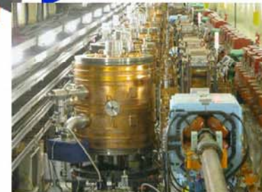
The state-of-art ARES copper cavities will be upgraded with higher energy storage ratio to support higher current.
