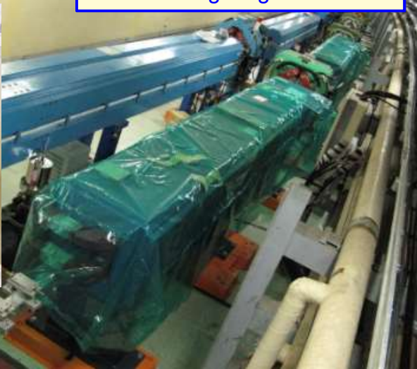
Installation of 100 new long LER bending magnets
