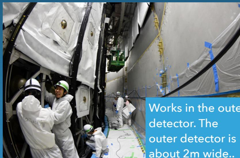
Works in the outer detector. The outer detector is about 2m wide..
